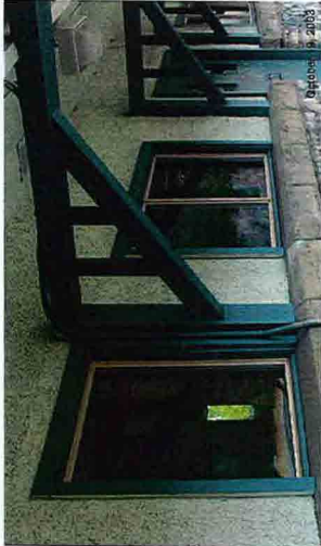
IMAGE NO.: 3-37 NORTH ELEVATION WINDOWS - Aluminum/ vinyl windows to be removed, new wood windows matching original window configurations to be installed.
