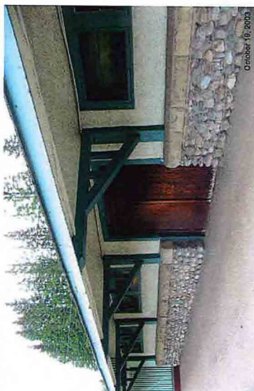
IMAGE NO.: 3-39 EXISTING WINDOWS ON NORTHEAST UPPER WINDOWS ORGANIZED HORIZONTALLY IN PAIRS - Windows to be maintained. - Door to be replaced with half-lite door.
