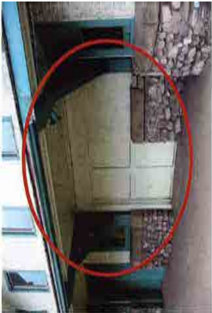
IMAGE NO.: 3-03 NORTH CENTRAL WALL EAST OF BAY - Re-instate original openings. - Retain cutstone sill. - Remove previous stone infill. - New stone base to match existing.
