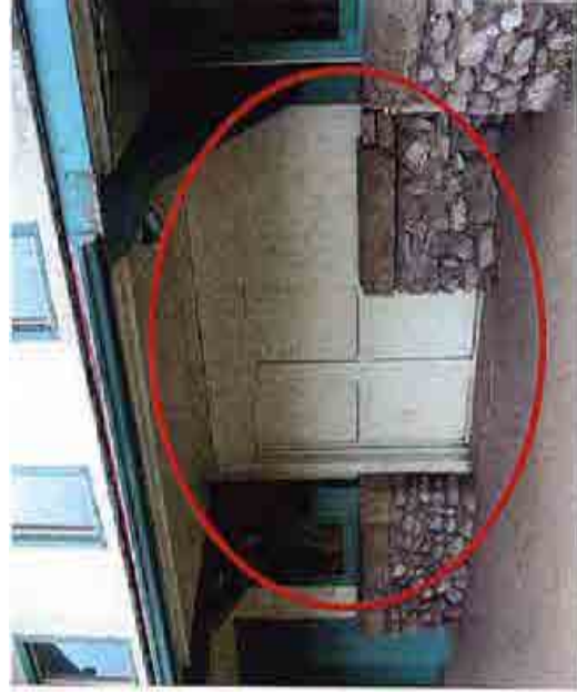
IMAGE NO.: 3-07 NORTH CENTRAL WALL EAST OF BAY - Re-instate original openings. - Retain cutstone sill for re-use. - Remove previous stone infill. - New stone base and cutstone sills to match existing.
