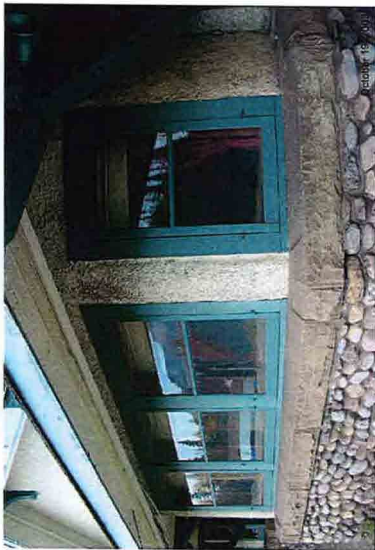
IMAGE NO.: 3-36 NORTH CENTRAL BAY LOWER WINDOWS WITH EXISTING STORM WINDOWS - Windows to be maintained.
