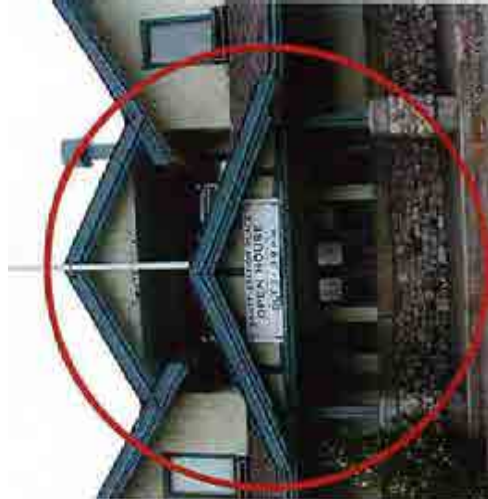
IMAGE NO. : 3-33 SOUTH CENTRAL - EXISTING BAY WINDOW - Remove existing bay window and stonebase. Retain cut sandstone sills and fieldstones for re-use. - Re-instate entrance with two side 6 pane windows. - Re-instate original window to east & west of main entrance. - Remove decorative fascia lighting. - Install new brackets to upper eaves. - Remove second floor planter boxes.
