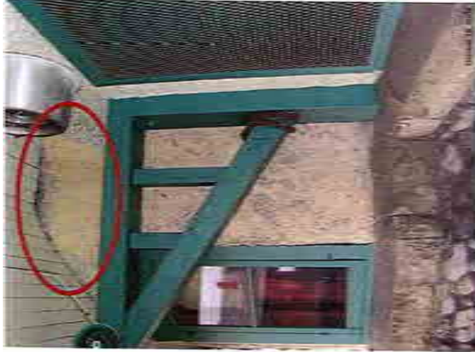
IMAGE NO.: 3-28 WEST SIDE OF NORTH BAY WINDOW - Remove speaker. - Remove kitchen exhaust fan. - Repair stucco to match existing. - Replace and install stucco to match existing when badly damaged or at new infills.
