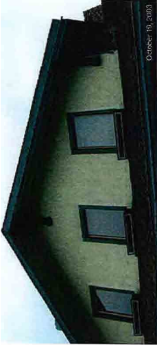
IMAGE NO.: 3-35 VIEW OF SOUTHEAST UPPER GABLE - Replace existing aluminum and vinyl windows with wood windows sympathetic to the original windows.
