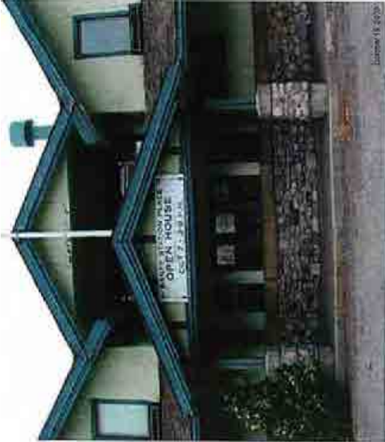
IMAGE NO.: 3-02 SOUTH VIEW OF ORIGINAL ENTRANCE AREA - Remove bay window addition installed 1973-1977. - Retain cutstone sills and fieldstone for re-use. - Re- establish original entrance location. - New stone base to match existing.
