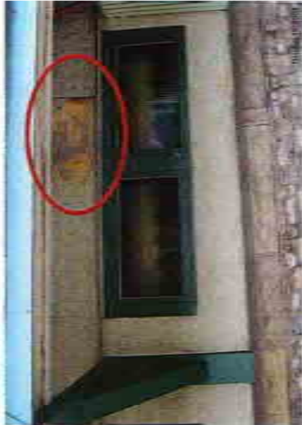
IMAGE NO.: 3-30 NORTHEAST WINDOW - Repair stucco to match existing. - Replace and install stucco to match existing when badly damaged or at new infills.
