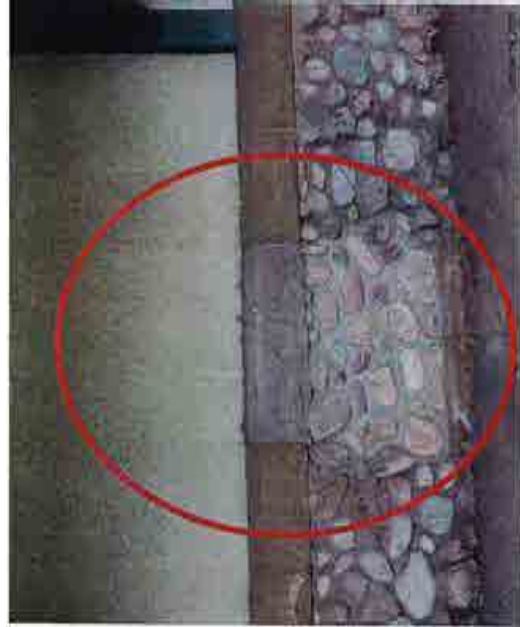
IMAGE NO.: 3-06 VIEW OF SOUTHWEST DOOR INFILL - Concrete sill to be replaced with a new sandstone sill to match existing. - Mortar to be re-pointed to match existing.
