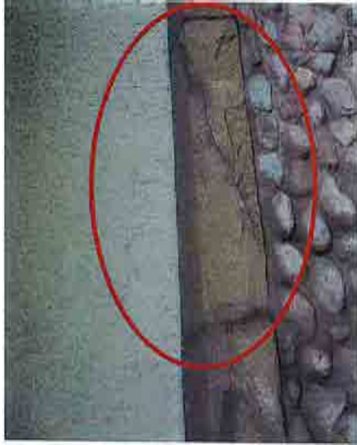
IMAGE NO.: 3-04 SOUTHWEST SILL CRACKED BUT APPEARS STABLE
