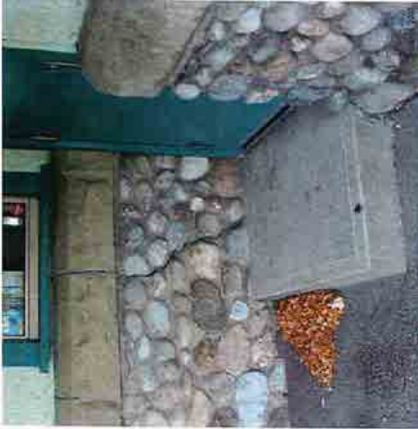
IMAGE NO.: 3-01 SOUTHWEST WALL AT EXIT STAIR - Repair and re-point mortar. - Window above to be infilled to satisfy exit separation. Stucco to match existing.
