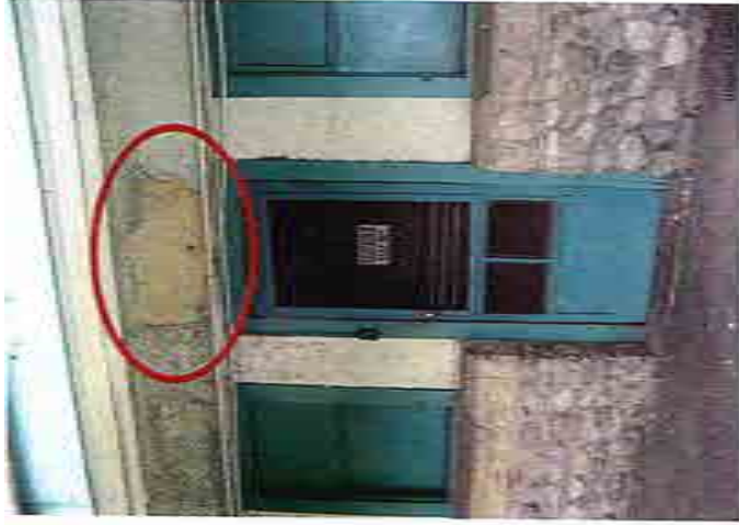
IMAGE NO.: 3-28 WEST SIDE OF NORTH BAY WINDOW - Remove speaker. - Remove kitchen exhaust fan. - Repair stucco to match existing. - Replace and install stucco to match existing when badly damaged or at new infills.
