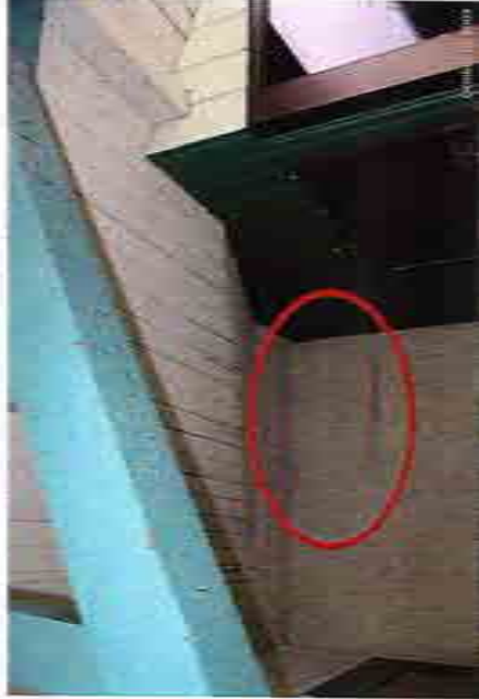
IMAGE NO.: 3-30 NORTHEAST WINDOW - Repair stucco to match existing. - Replace and install stucco to match existing when badly damaged or at new infills.
